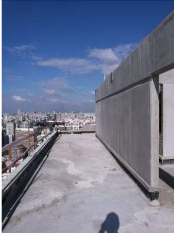
Torre Arcos – Contrapiso Remate
