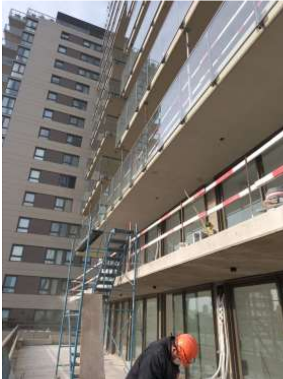
Piso 11°. Retiro Defensas s/Arcos
